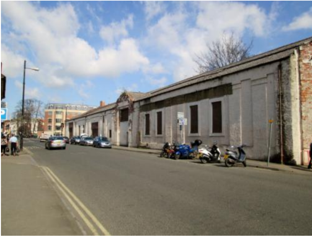
Photograph No. 1 – Piccadilly elevation
