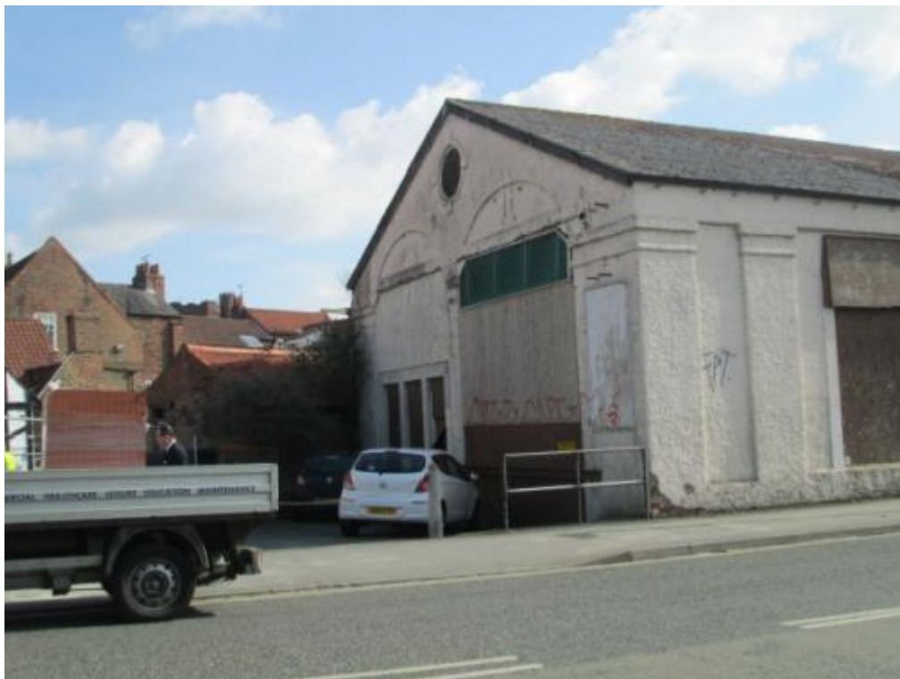
Photograph No. 4 – North West elevation
