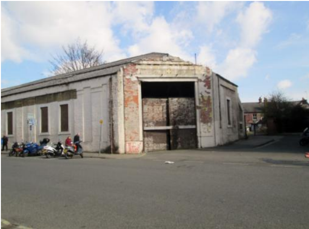
Photograph No. 3 – Dennis Street elevation
