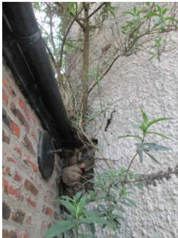
Photograph No. 29a – Rear corner of North West elevation
