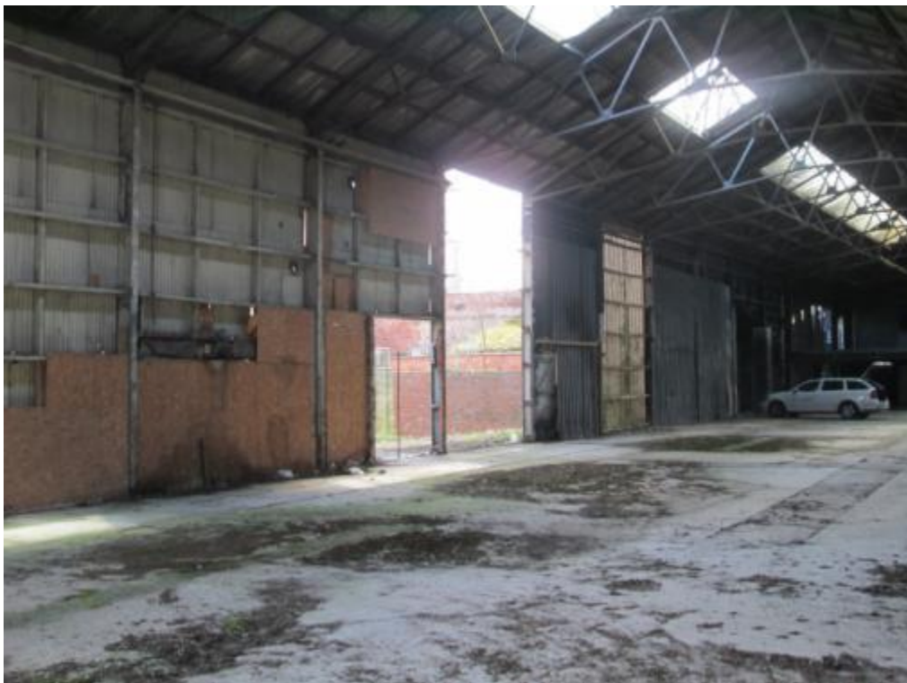
Photograph 41 – Part view on rear elevation
