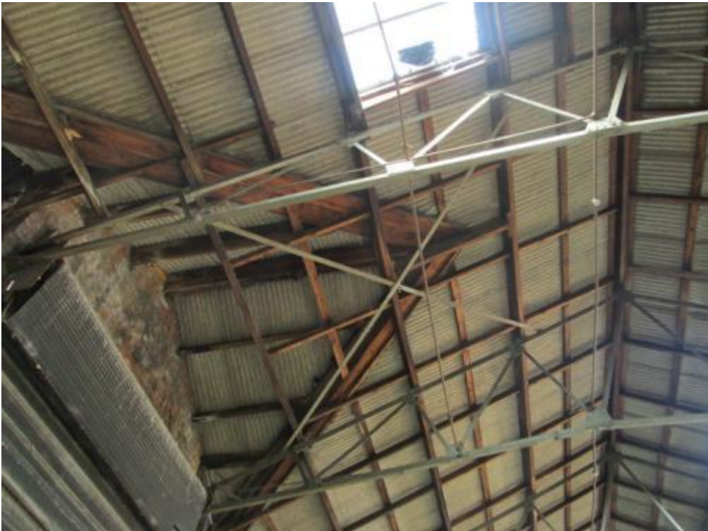
Photograph 52 – Cross bracing in roof
