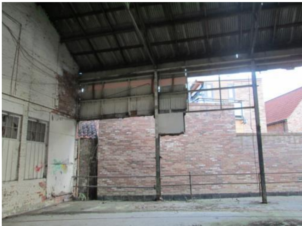
Photograph 39 – Part view on rear elevation
