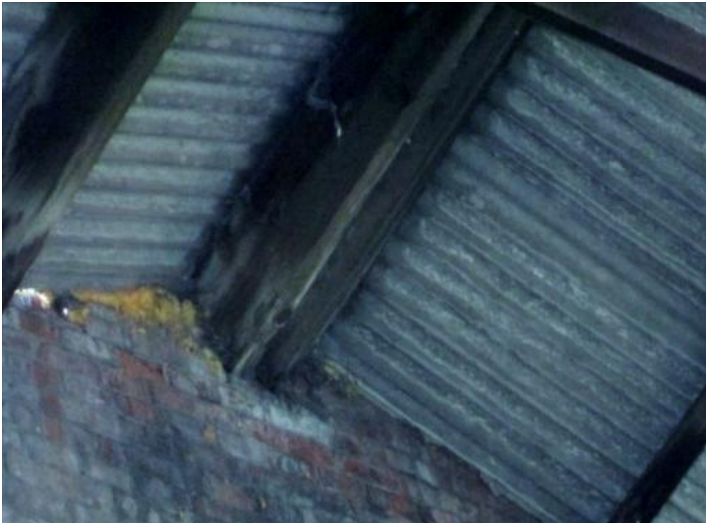
Photograph 49 – Purlins bearing into wall above Piccadilly entrance
