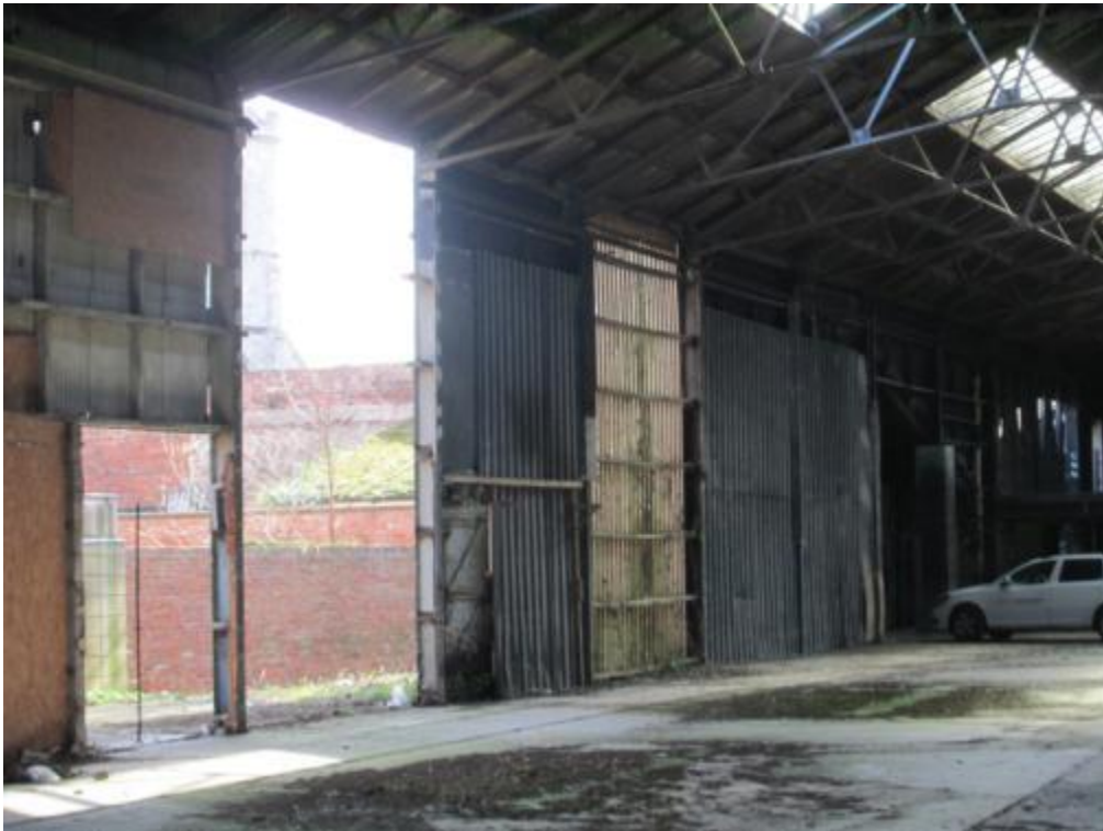
Photograph 41a – Part view on rear elevation
