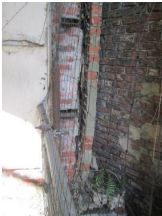
Photograph 71 – Internal view of North West elevation rear corner
