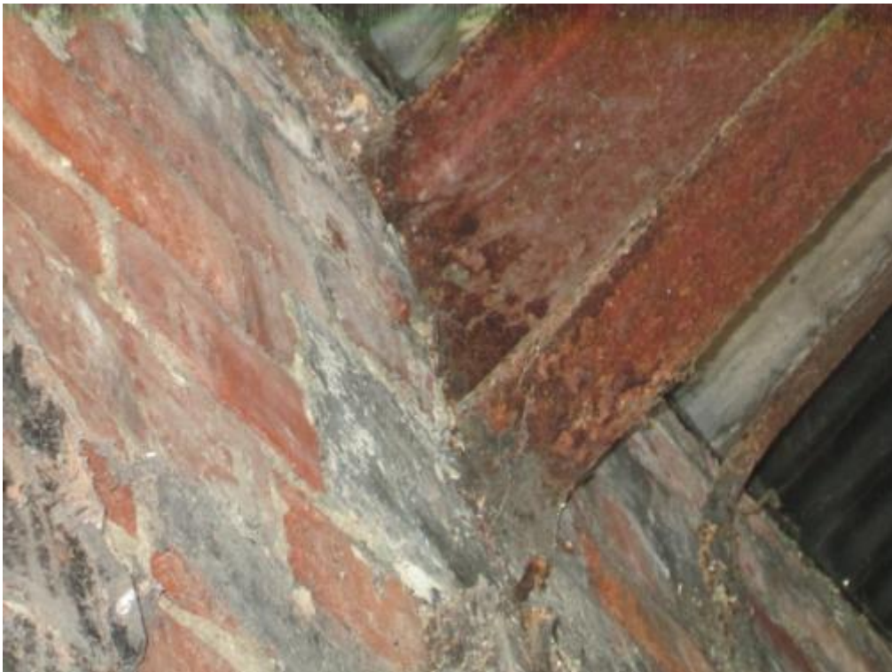
Photograph 67 – Steel rafter over lean-to bearing on external wall
