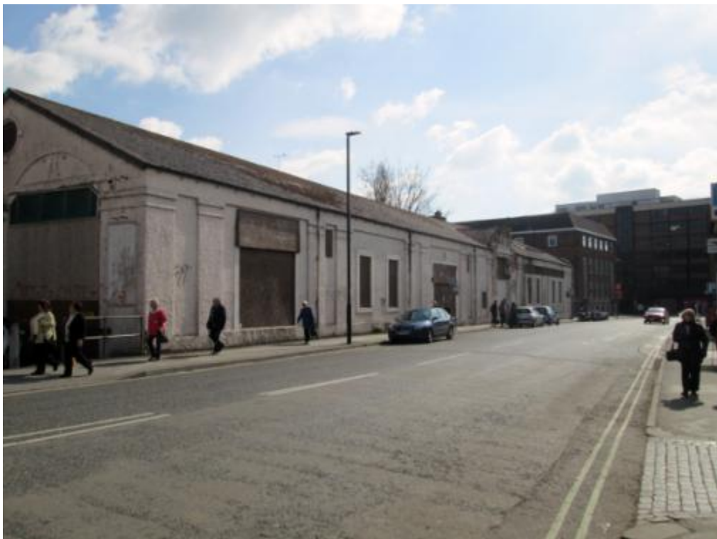
Photograph No. 2 – Piccadilly elevation
