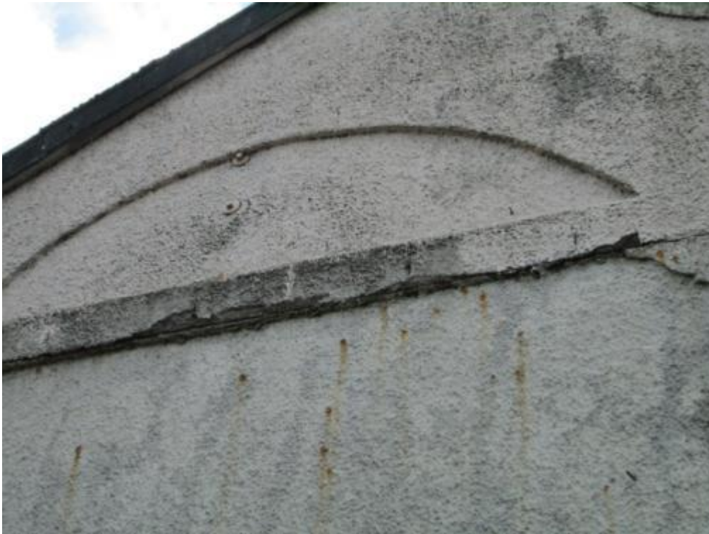
Photograph No. 27– Part North West elevation
