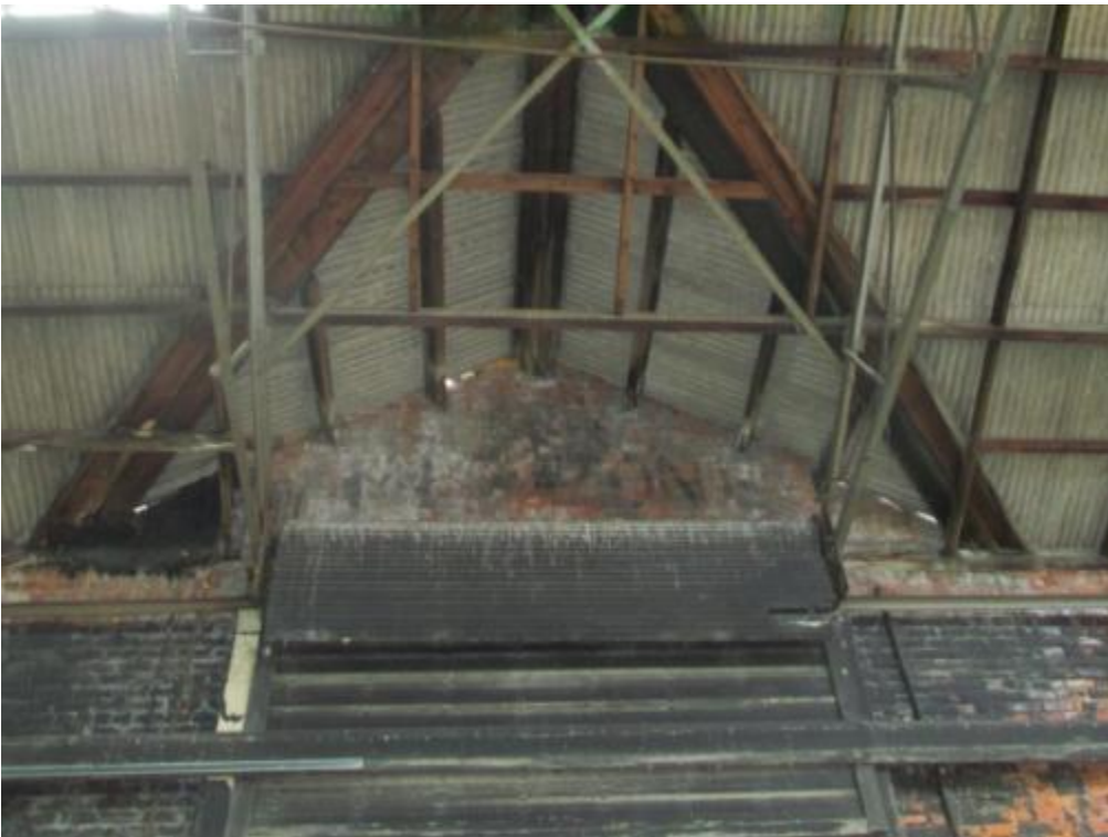
Photograph No. 36 – Internal view above Piccadilly entrance
