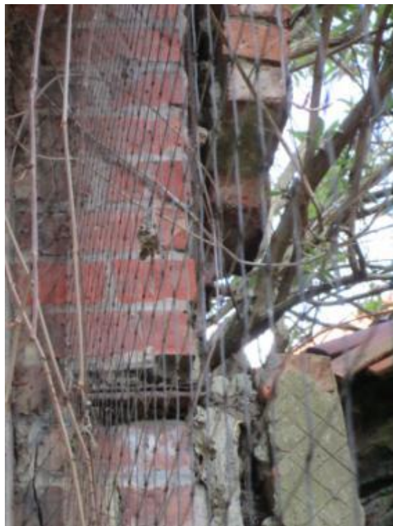
Photograph 73 – Internal view of North West elevation rear corner
