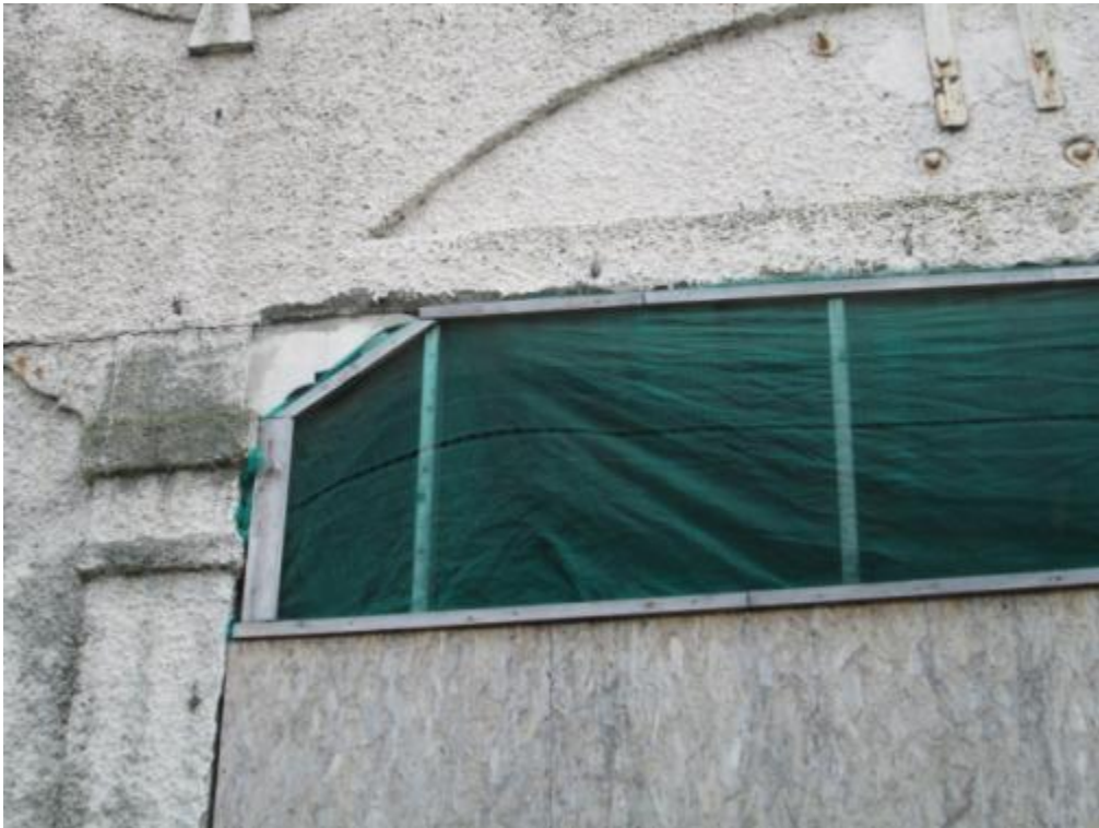
Photograph No. 25 – Part North West elevation
