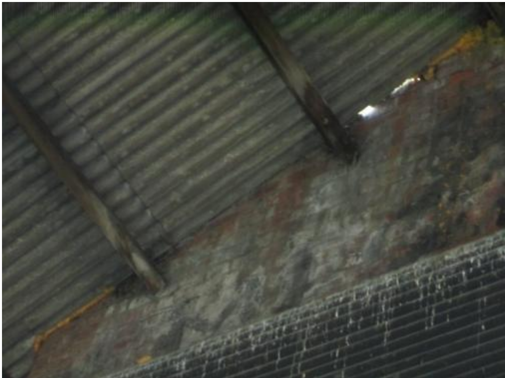
Photograph 49-50 - Purlins bearing into wall above Piccadilly entrance
