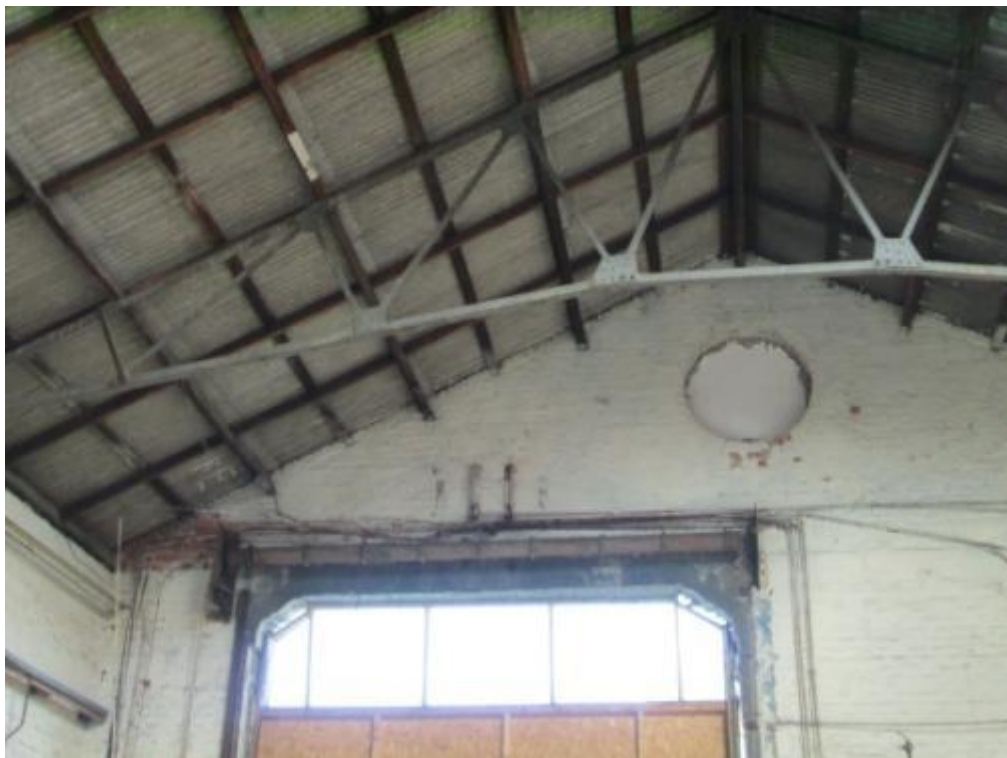
Photograph 37 – Internal view towards North West entrance
