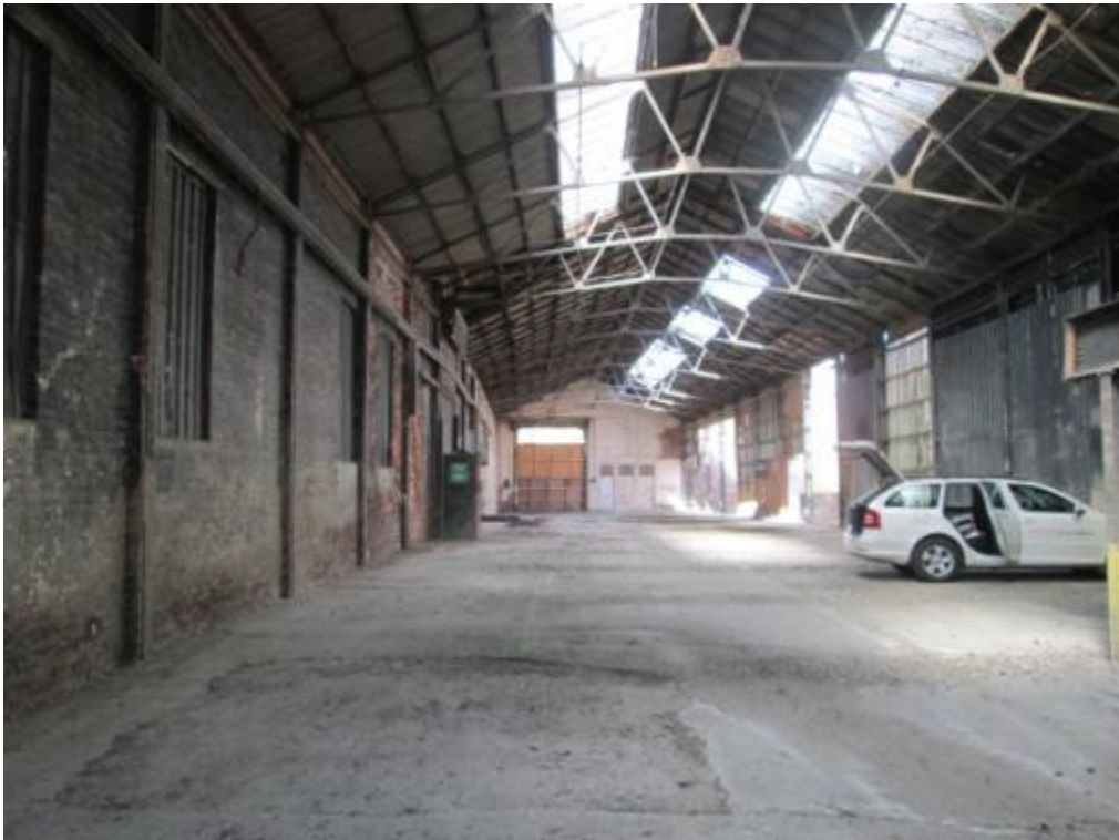
Photograph 61 – Internal view from Dennis Street
