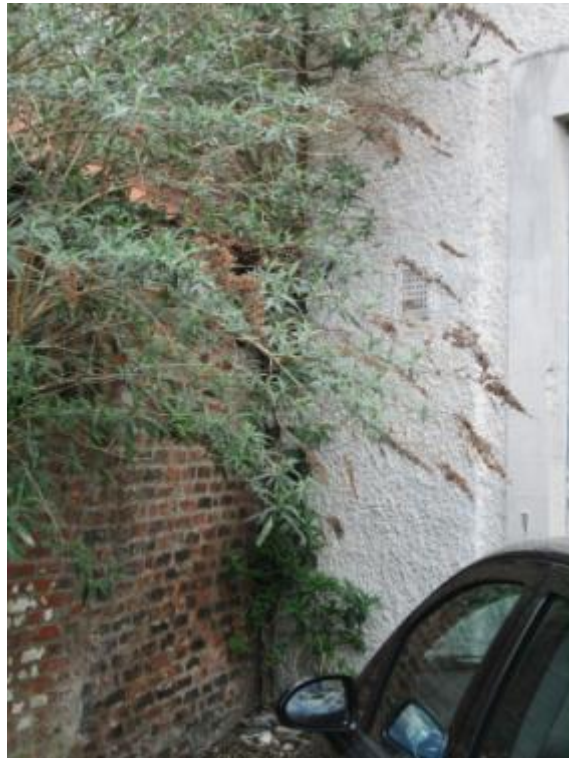
Photograph No. 29 – Rear corner of North West elevation
