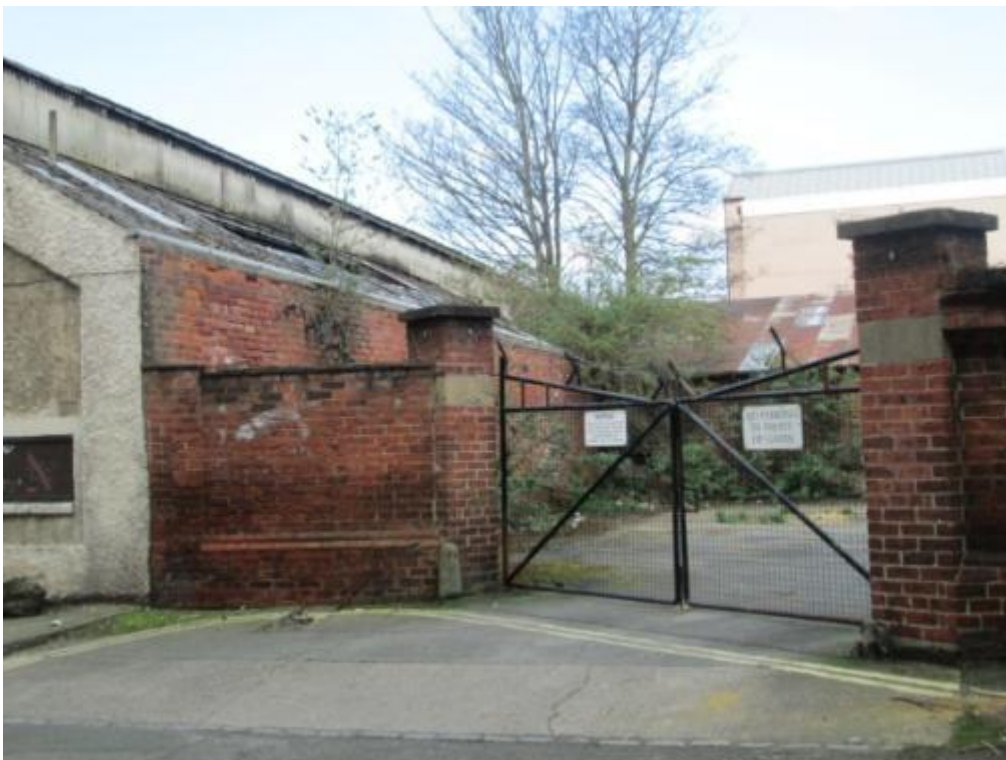
Photograph No. 33 – Rear elevation
