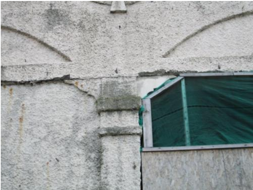
Photograph No. 26 – Part North West elevation
