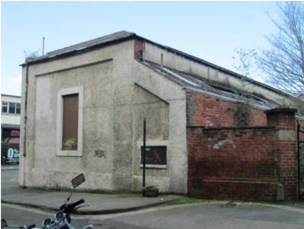
Photograph No. 32 – Dennis Street elevation
