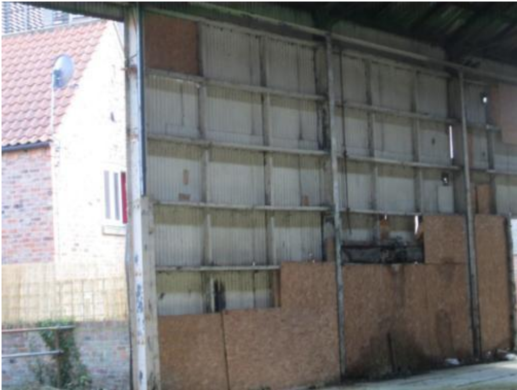
Photograph 40 – Part view on rear elevation
