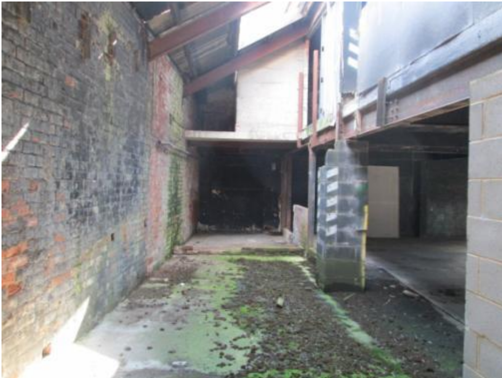
Photograph 63 – Internal view within lean-to looking towards Dennis Street end
