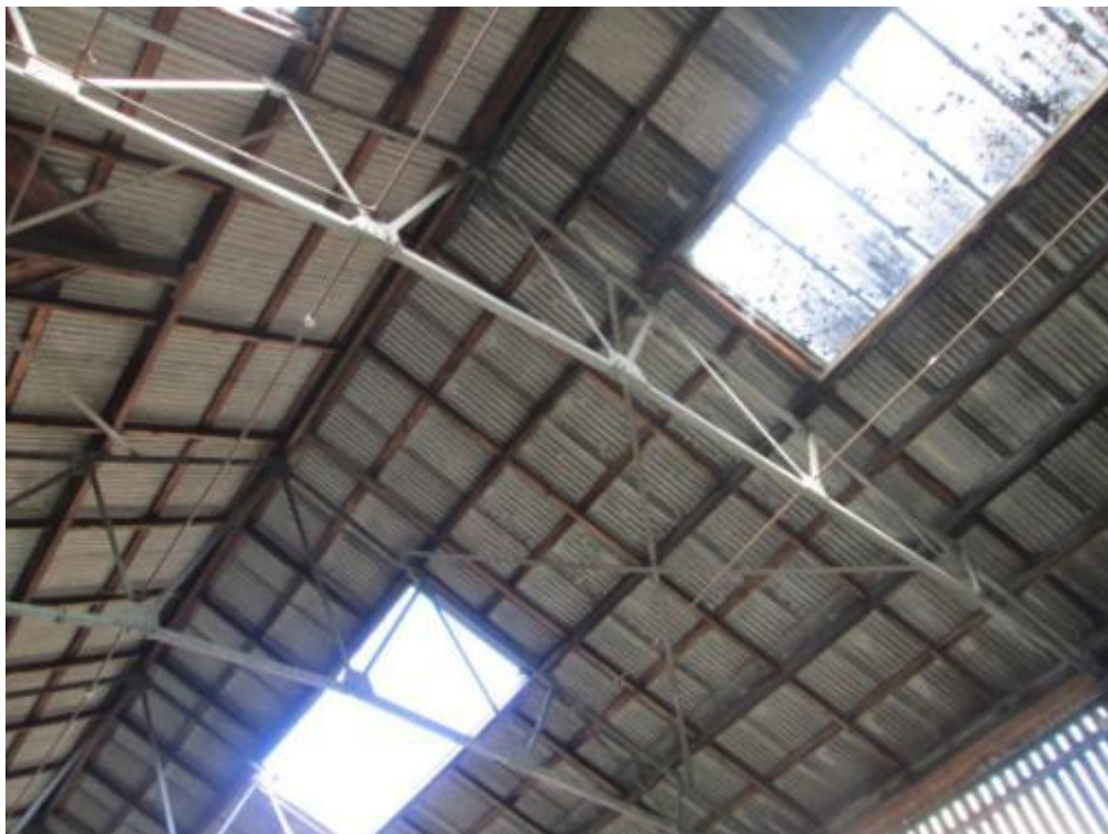
Photograph 53 – Cross bracing in roof
