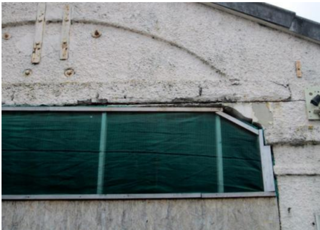
Photograph No. 24 – Part North West elevation
