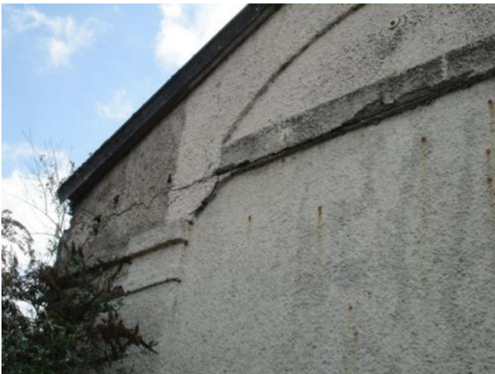
Photograph No. 28 – Part North West elevation
