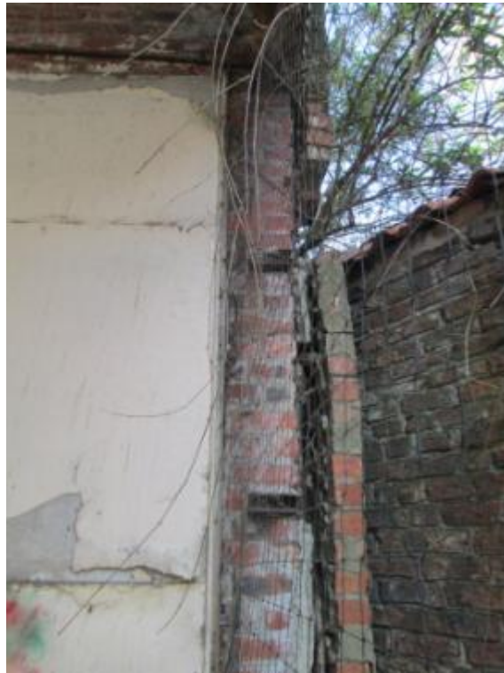
Photograph 72 – Internal view of North West elevation rear corner
