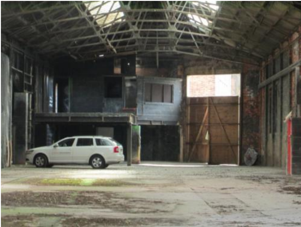
Photograph 59 – Internal view towards Denis Street
