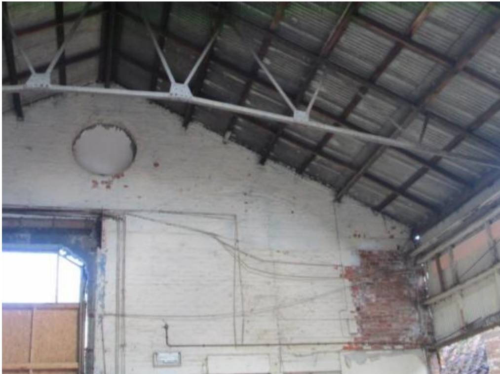
Photograph 38 – Internal view towards North West entrance
