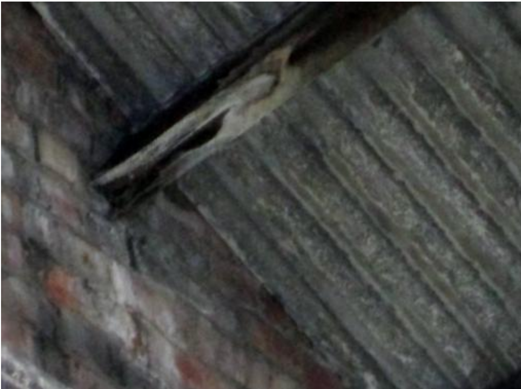
Photograph 47 – Purlin bearing into wall above Piccadilly entrance
