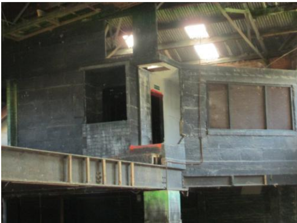
Photograph 42 – Partially demolished wall at Dennis Street
